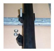
Locate the other half of the cable clamp. Secure with a nut and washer (not supplied) to the support structure and tighten.
