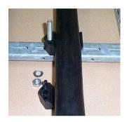
3) Locate the other half of the cable clamp. Secure with a nut and washer (not supplied) to the support structure and tighten.
