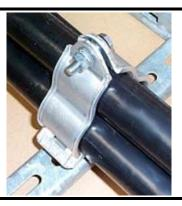
**NOTE:** Do not over-tighten. The cleat should secure the cable but does not need to be so tight that the cable bulges at either side of the cleat.
