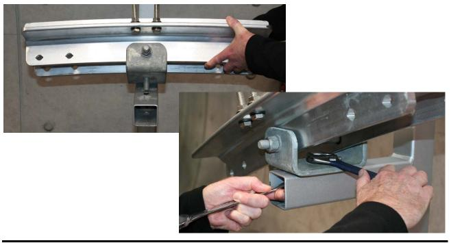
2) With care install the cable into the saddle.
