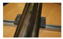
Fit the top half of the cleat over the cables. Secure with the M12 setscrews and flange nuts (19mm spanner/socket for setscrews, 16mm spanner/socket for flange nuts).
