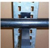
3) Locate the retaining strap through the aperture at the rear of the cable support, hand tighten.
