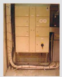
AFUMEX LSX<sup>™</sup> is lightweight and compact in design, allowing cost savings to be made by the selection of smaller, lighter ⊠xings, supports and cable tray or basket. AFUMEX LSX<sup>™</sup> is also quick to install and easily stripped, signi⊠cantly reducing the ⊠rst and second ⊠x termination times when compared with SWA cable (Steel Wire Armoured).
