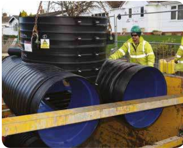
Pre-fabricated Ridgistorm-XL solution chosen for Welsh Water capital works scheme
