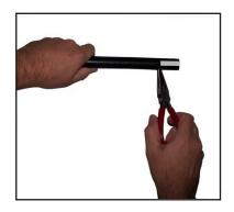
Peel scored semi-con segments with needle nose pliers or other suitable tool. Perfectly scored semi-con is cleanly removed without damage to underlying insulation.
