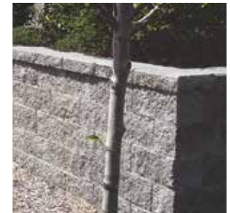
Keystone retaining wall in Flint finish
