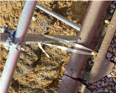
Simple installation of temporary safety railings
