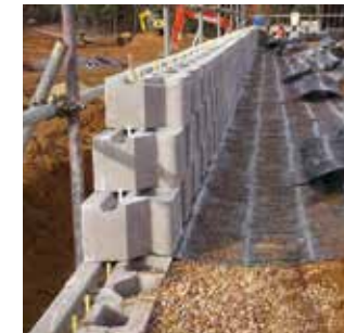
Keystone during construction
