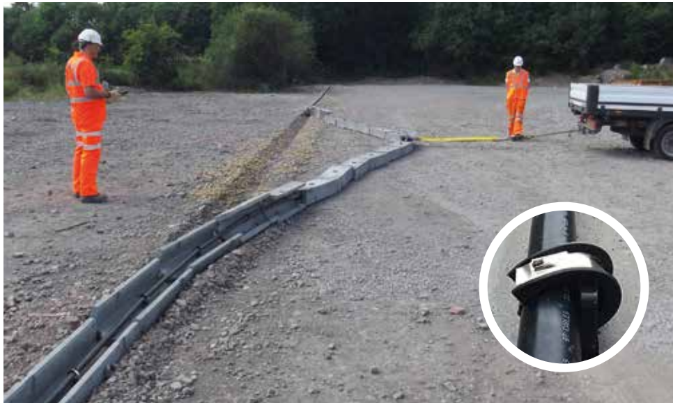
Maximum disruption of vehicular cable pull
