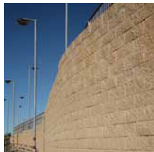
Railway station walls
