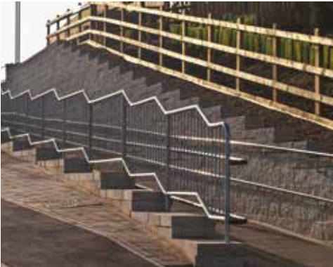
Keystone retaining wall
