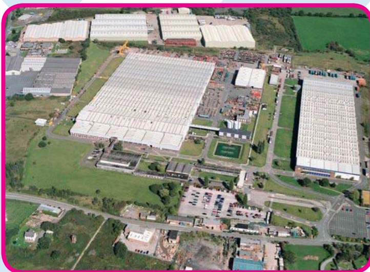
Prysmian Plant - Wrexham
