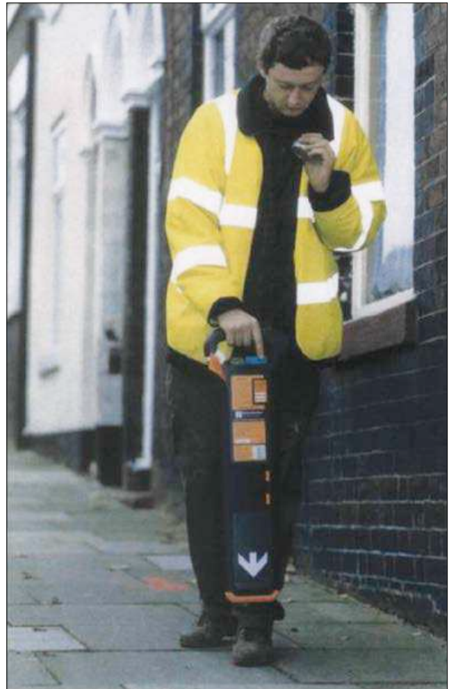
Figure 5 Using a cable locator
