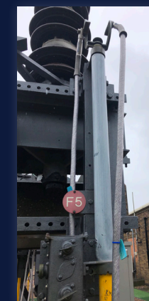
Substation Fixed Earthing
