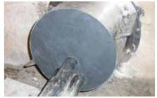
After the frame has been installed, the RISE Duct sealing system can be applied. The depth of the frames is 80mm which accomodates 60mm insert and filler sleeves. The remaining 20mm is used for applying a 20mm layer of sealant.
