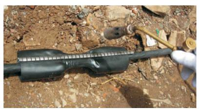
Used extensively worldwide to provide the outer protection and sealing of telecommunication cables, they are equally useful for power cable joint outer sealing reducing trench excavation.
