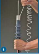
8. Shrink into place by unwinding the removable core.
