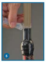
5. Apply a liberal bead of silicone lubricant to the semi-con shield step.
