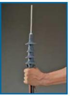
9. Apply silicone lubricant to skirt and mastic area.
