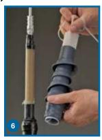
6. Pull the loose end of the core cord until the core is even with the end of the termination housing.
