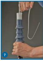
7. Position the terminator onto the cable.
