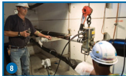
8 Join the conductor using a compression, welded or other type of connector.
