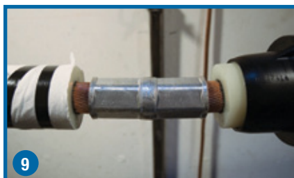
9 Conductors shown joined using a compression connector.
