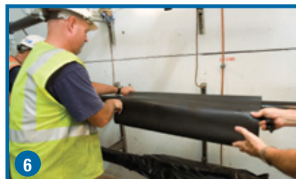
6 Store the cover-up sleeve on each cable.
