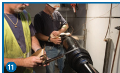
11 Seal joint ends with mastic wrap.
