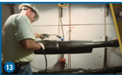
13 Position and shrink cover-ups.
