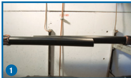
1 Overlap cables, straighten and strip back jacket.
