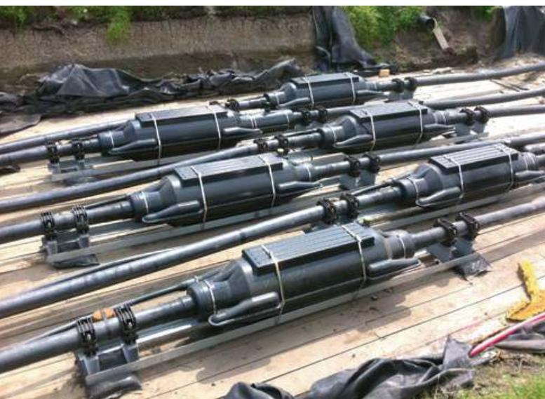
Crossbonding joints / Crossbondingmuffen
