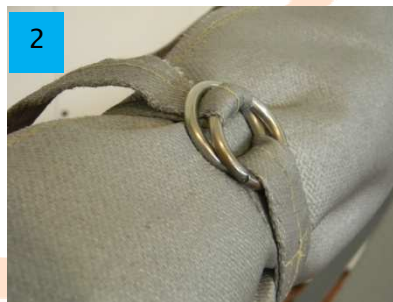
WRAP THE COVER AROUND THE JOINT
