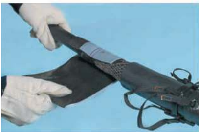
Applying sealing mastic
