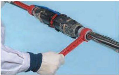
Breaking the internal connection of the support tube
