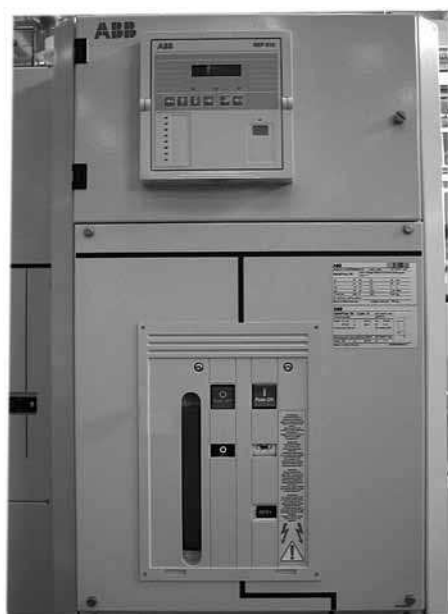
V-module with protection relay type REF610 in integrated LV-compartment with hinged door
