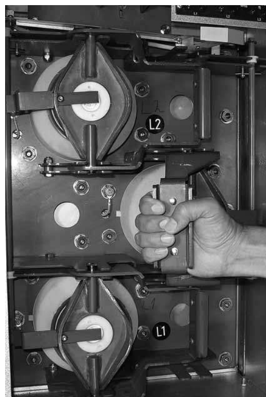
4. Pull handle and open the fuse canister.
