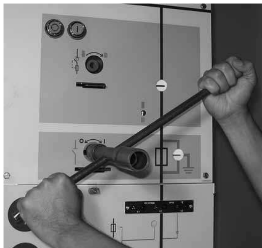
2. Close earthing switch by turning operating handle clockwise..
