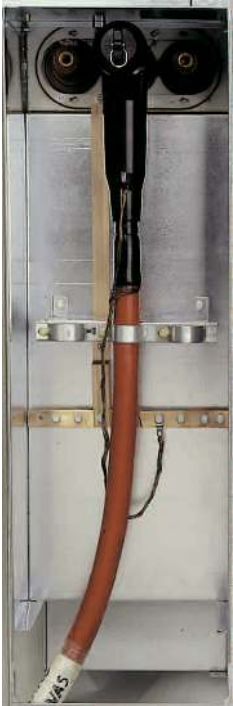
Connection. EUROMOLD screw-in T-terminal (K-400TB)
