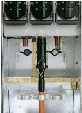
Connection. EUROMOLD straight plug-in terminal (K-152SR)
