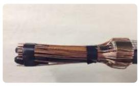
• Form the neutral earth wires back over the phase cores and cut to length if required.
