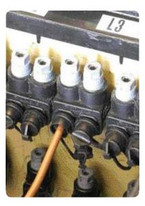
• Tighten the 13mm head of the phase connector (Section 4.2.3).
