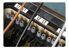
• Cut the core to length and remove 15mm or core insulation (Section 3.6.4).
