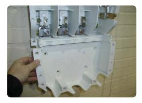
• Once the cut-out is mounted offer the cable up against the cut-out and cut it to length, so it overlaps the top of the cut-out by approximately 50mm.
