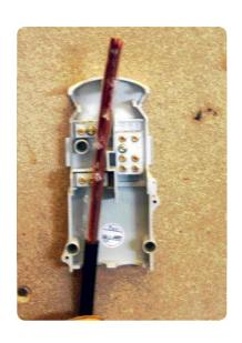
• Prepare the copper neutral earth wires (Section 3.5.2). Set the phase and neutral conductors so that they line up with the terminal in the cut-out to be used.
