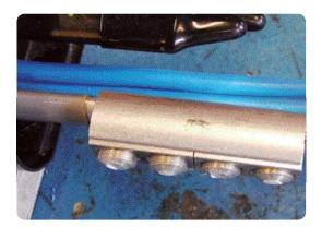
• Insulate the mechanical phase connectors with the piece of CR sheet insulation (Section 4.9.4).
