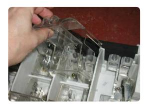
Place screening and internal components in a safe location where they will not be lost or damaged. Mount the cut-out on to the required surface with suitably sized screws. The top two fixings
