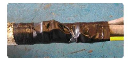
• Cut one of the 'live' phase cores to length (Section 3.2.8) and remove the paper insulation (Section 3.2.9).
