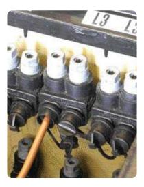
• Tighten the 13mm head of the phase connector (Section 4.2.3).
