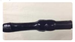
• Shrink the large heatshrink tube over the end of the joint, starting from the earth braid and working towards the cable end (Section 4.10.2).
