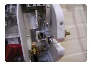
• Re-tighten the two retaining screws in position and replace screening.
