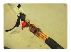
Bend the CNE wires back over the outer sheath of the cable and secure in place with PVC tape.
