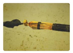
Carefully cut the CNE wires next to the mechanical connector connecting them to the external earth wire, if fitted.
