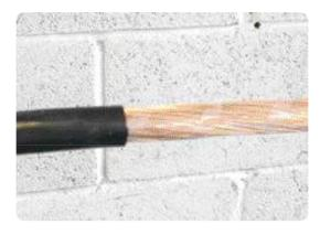
• Unwind the copper neutral earth wires and temporarily fold back along the cable sheath.
