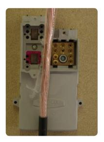
• Prepare the copper neutral earth wires (Section 3.5.2). Set the phase and neutral conductors so that they line up with the terminal in the cut-out to be used. Remove any plugs in the cut-out.
