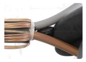
• Pull the 3-Phase cores back together and apply two layers of black moisture-sealing mastic around them next to the copper wires.
