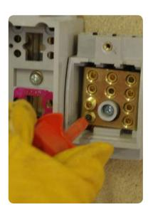
Install the crutch cover and fix in place with the screws provided.
