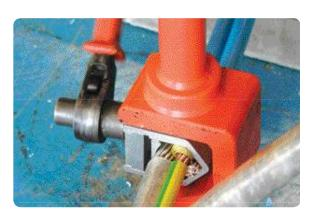
• Insulate the US3 connector with the piece of CR sheet insulation (Section 4.9.4).
