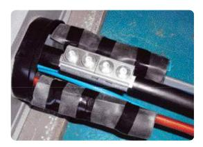
• Cut the neutral earth conductors to length on both the link box and the cable tail, so that they overlap sufficiently to enable the brass CNE shear-bolt connector to be installed, as shown in the diagram below. Install the mechanical brass connector in the position indicated and shear off (Section 4.1.3).
