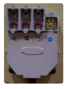
• Install the plastic cover for the neutral earth block and secure in place with the screw provided.
