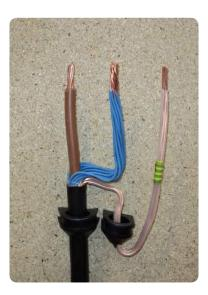
• Insert the correct conductors into the correct terminals of the cut-out and tighten the Allen screws with an approved insulated Allen key tool. Ensure that the conductors are completely installed under both screws of each terminal.
