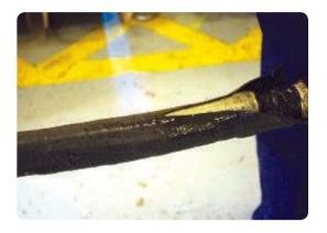
Carefully unwind and remove the layer of tinned copper mesh tape.
