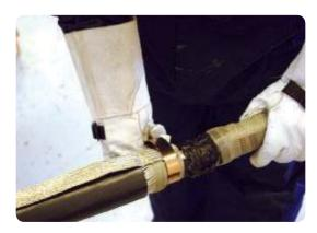
• Unwrap and remove the constant force spring around the neutral earth braid.
