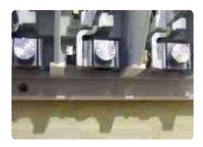
Position and secure the cable trough using the four screw points provided.
