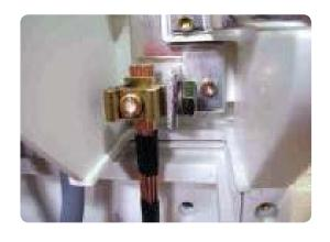
• Re-install all phase barriers, phase stalk shrouds, rubber grommets and the cable entry board in to the cut out.
