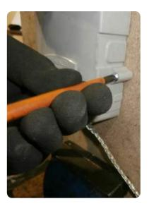
• Install the "Consumers Earth Connection" label onto the tinned copper braid.
