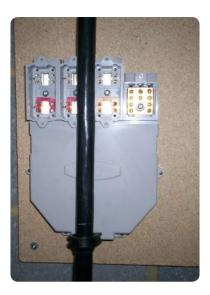
• Mark the removal point of the PVC sheath, so that it is at least 20mm inside the cable crutch cover. Remove the PVC sheath (Section 3.6.1).
