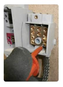
• Install the crutch cover and fix in place with the screws provided. Ensure that the tinned cooper braid from the neutral earth block is positioned so it comes out of the right hand cable entry in the crutch cover and install the cover using the screws provided.
