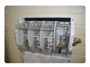
Install the cable sealing chamber cover and the red incoming phase shrouds.
