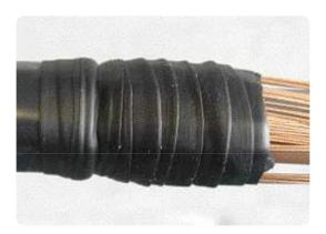
Apply two half-lap layers of PVC tape over the mastic under tension. The PVC tape should extend either side of the black moisture-sealing mastic tape.
