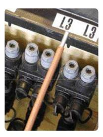
• Insert the phase conductor into the required phase connector.
