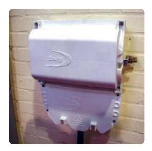
• Install screw guards and seal with an approved meter sealing device. Six screw guards are provided one for each of the screws on the cut-out lid and two for the cable trough.
