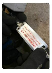
• Install the earth block onto the end of the tinned copper braid and fix the earth block onto the meter board next to the crutch cover of the cut-out.
