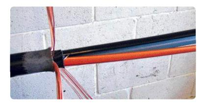
Temporarily tape all the cores together with PVC tape.
