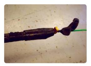
Remove the section of PVC sheath from the body of the joint.
