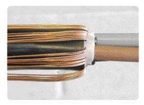
• Separate the 3-Phase conductors allowing sufficient space to insert the black moisturesealing mastic.
