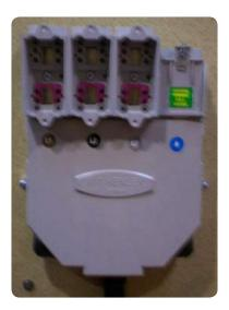
• Push the fuse carriers into place and seal with an approved meter sealing device.
