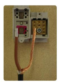
• Insert the correct conductors into the correct terminals of the cut-out and tighten the Allen screws with an approved insulated Allen key tool. Ensure that the conductors are completely installed under both screws of each terminal.
