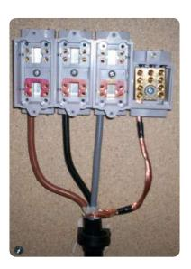
• Insert one end of the tinned copper braid from the PILC cable earth bond kit into the bottom right hand terminal of the neutral earth block and tighten the Allen screws with an approved insulated Allen key tool. Ensure that the conductors are completely installed under both screws of each terminal.
