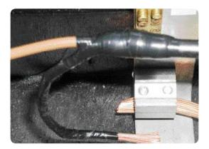
Perform an insulation resistance test on the service cable.
