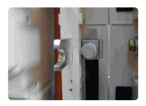
• Install all 3-Phase conductors into the mechanical phase connectors and shear off (Section 4.6.1).
