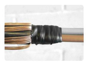
• Neatly lay the copper wires back over the mastic tape, ensuring that the wires do not cross.
