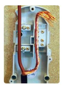
• Cut the phase and neutral conductors to the length required for the terminals to be used in the cut-out.
