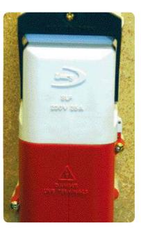
• Fix appropriate phase identification (L1, L2, L3 and N) labels to the cut-out.
