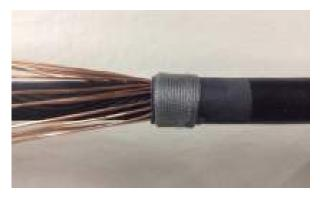
• Wrap the tinned copper mesh around the cable sheath next to the sheath cut.
