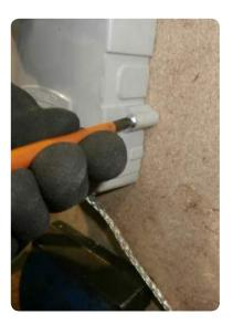
• Install the "Consumers Earth Connection" label onto the tinned copper braid.
