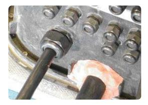
Remove the PVC oversheath from the service cable (Section 3.6.1).
