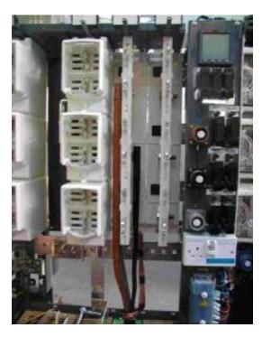
• Install the neutral conductor into the mechanical neutral earth connector and shear off (Section 4.1.1).
