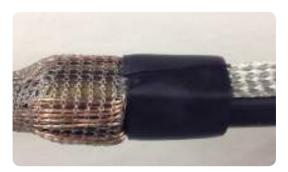
Apply the black mastic tape around the abraded exposed cable sheath behing the constant force spring. Starting underneath the braid before continuing around the braid, ensuring that the braid is completely covered.
