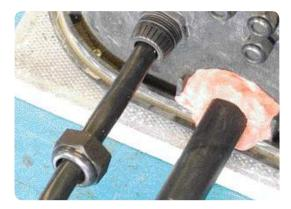
Screw the gland cap onto the gland and tighten down on to the cable.
