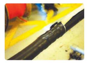
• Pull the hot sleeve off of the joint completely.
