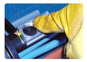
• Install all three mechanical straight connectors on to the cable stubs on the link box (Section 4.3.1).
