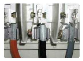
• Install all three phase conductors into the mechanical phase connectors and shear off, as described in Section 4.6.1.
