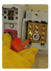
Insert one end of the tinned copper braid from the PILC cable earth bond kit into the bottom
