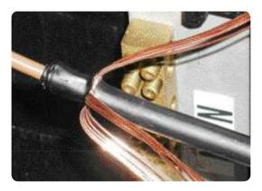
• Neatly lay the copper wires back over the mastic tape, ensuring that the wires do not cross.
