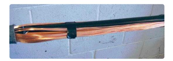
• Position the distribution unit over the cable, by inserting the cable through the hole provided. Ensure that the abraded section of cable oversheath is fully inside the unit.
