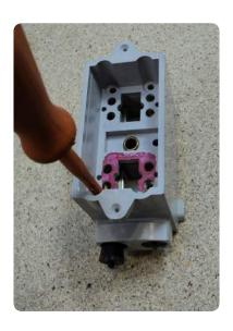
• Offer the cable up against the cutout and cut it to length, so that it overlaps the top of the cut-out by approximately 50mm. Cut one of the rubber grommets to match the outside diameter of the cable, pass it over the cable and park it below the cut-out.
