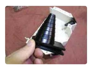
• Cut out the centre of one of the supplied grommets to match the diameter of the cable to be installed. Slide it down over the cable, so it can be easily installed.
