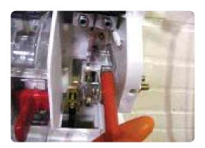
• Remove the split link and reposition in the in the position shown.
