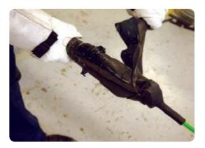
• With the inner heat shrink cap still cold score the surface of the tube, with an approved knife, over the area where it overlaps the PVC outer sheath and the CNE wires below.
