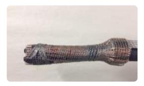
Apply one half lap layer of tinned copper mesh over the joint from the constatnt force spring to the end of the heatshrink end caps.
