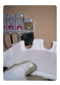
• Install the crutch cover and fix in place with the screws provided. Ensure that the tinned cooper braid from the neutral earth block is positioned so it comes out of the right hand cable entry in the crutch cover.
