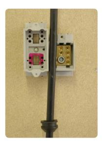
• Mark the removal point of the PVC sheath, so that it is at least 20mm inside the cable crutch cover. Remove the PVC sheath (Section 3.5.1).
