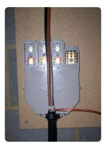
• Set the phase and neutral conductors so that they line up with the terminal in the cut-out to be used.
