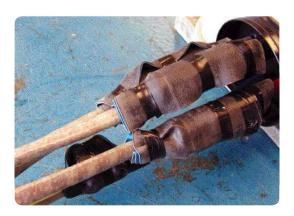
• Remove all temporary shrouding from the lead sheath and armours.
