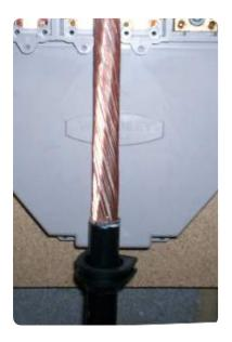
• Prepare the copper neutral earth wires (Section 3.6.2).
