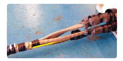
• Fit the two halves of the plastic joint shell (Section 4.8.1). Install metal clips and brown putty to ensure that JEM resin does not leak out when installed.
