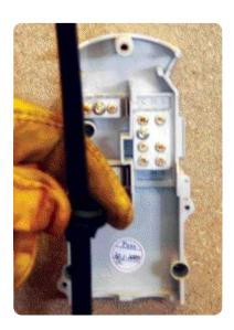
Mark the removal point of the PVC sheath so that it is at least 20mm inside the cable crutch cover. Remove the PVC sheath (Section 3.5.1).
