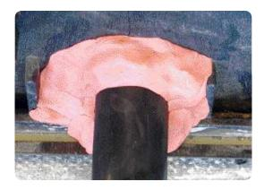
• Fill the unit with the correct amount of JEM resin as shown in the table at the start of this section, so that there is a minimum of 10mm coverage over all the mains connectors (Section 4.8.2).
