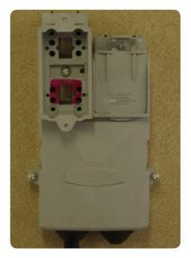
• Push the fuse carrier into place and seal with an approved meter sealing device.
