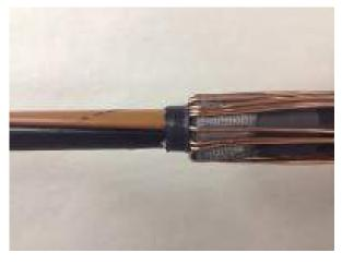
• Open out and clean the neutral/earth wires and fold back over the tinned copper mesh.
