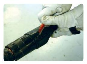
Apply sufficient heat to the cap so that the outer heatshrink tube starts to shrink, split and come away from the layers below.
