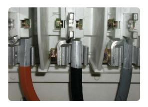
• Install all 3-Phase conductors into the mechanical phase connectors and shear off, as described in Section 4.6.1.
