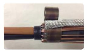
• Position the end of the earth braid with the solder block, over the neutral earth wires and the tinned copper mesh and fix in place with one turn of the supplied constant force spring.
