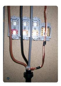
• Cut the phase and neutral conductors to the length required for the terminals to be used in the cut-out. Remove the insulation from the phase cores to the length required by the terminal in the cut-out (Section 3.6.3).
