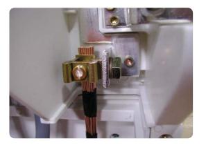
• Reinstall all phase barriers, phase stalk shrouds, rubber grommets and the cable entry board in to the cut-out.
