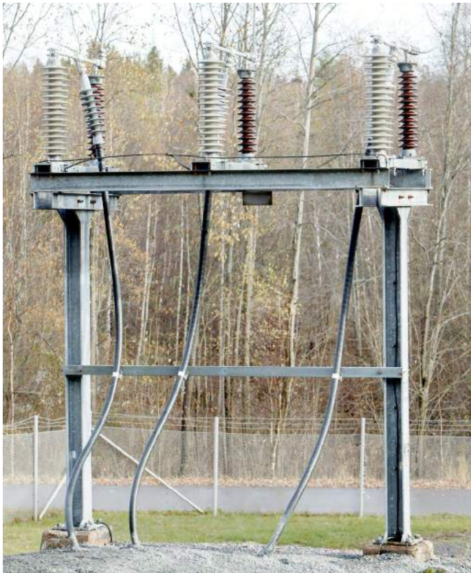
PEXLIM surge arresters protecting a cable entrance
