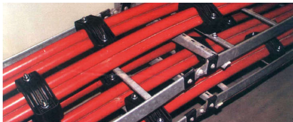
Replacement with id-Technik Cable Clamps: KP Series
