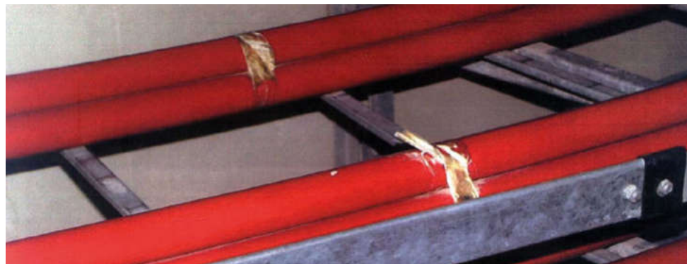
Bundling with fibre-glass reinforced bundling adhesive tapes, functional breakdown of the tapes due to ageing
