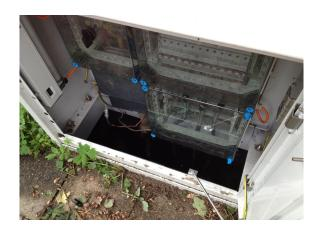
2 component sealant used to seal the base of street cabinets.
