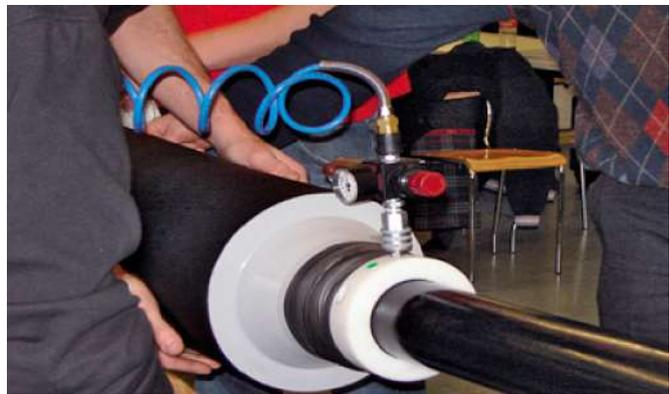
Assembling-friendly installation of a slip-on joint by "air cushion" method
