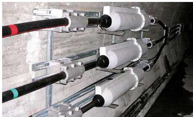
Joins with polyester protection box in a concrete tunnel
