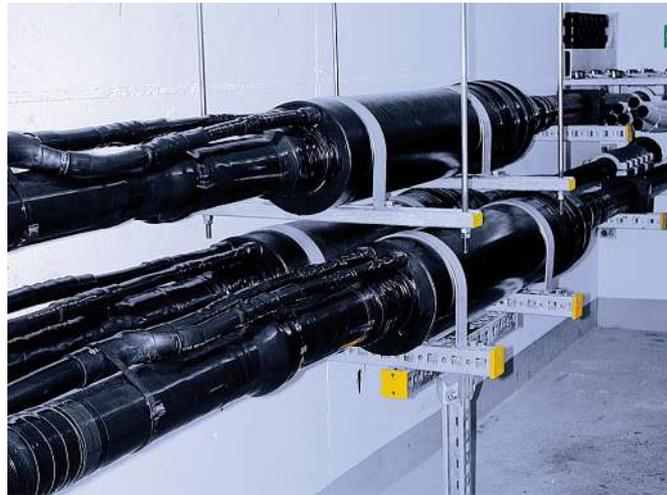
Joins with Cu-tube and HDPE coating in a concrete tunnel
