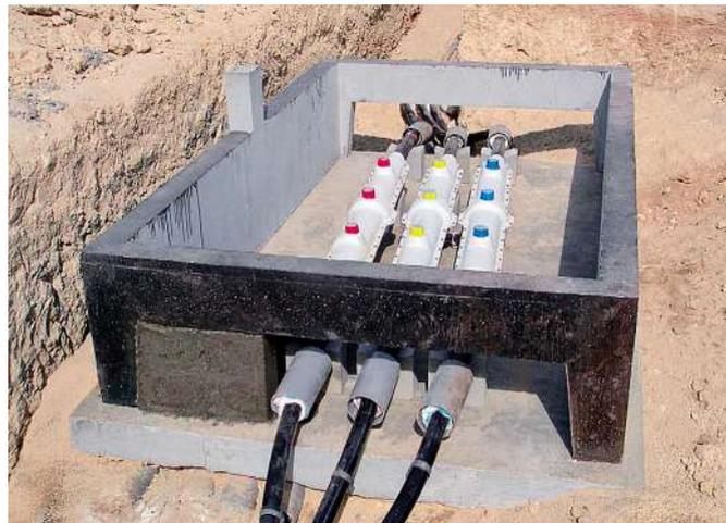
Joins with polyester protection box in a concrete pit
