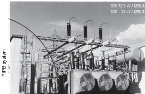
Figure 28.4(h) Layout of a 72.5 kV/1250A PIPB at a switchyard (Courtesy: MGC Technologie AG)
