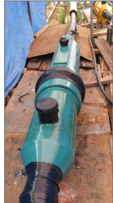
▲ Installation of premolded joint.
