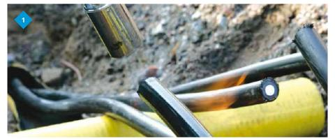
**Apply heat symmetrically**Use a mid-to-high flame to heat the outer sheath. Keep the flame moving all the time around the cable and through the whole peeling length.
