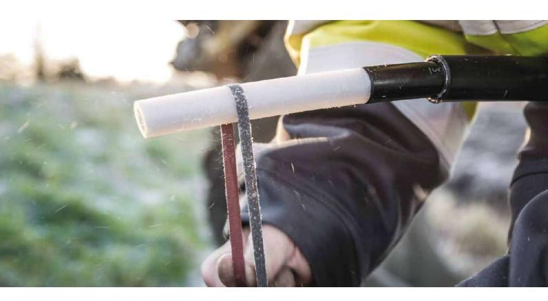
In most cases, faults that occur in cable accessories are the result of errors in cable preparation.
