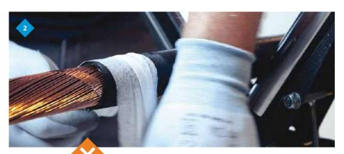
Always clean the outer sheath before removal and after grinding it.
