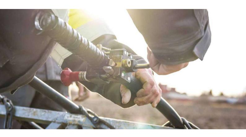
The metallic screen defines what tool can be used for removing the outer sheath.
