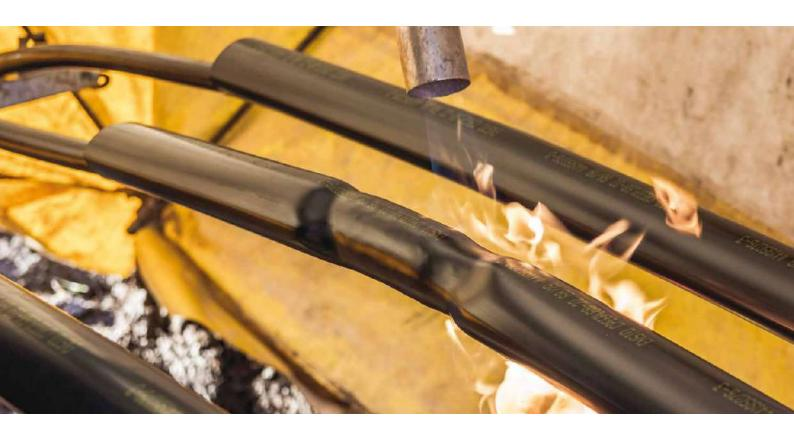
The mechanical robustness of heat-shrink accessories is the main advantage of the technology.
