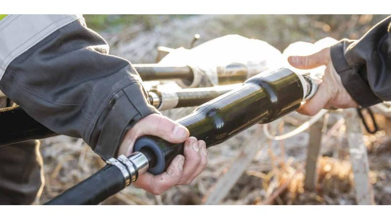
The reliability of several components integrated into one body and shorter installation times are the main advantages of cold-shrink and hybrid technologies.
