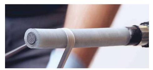
**Grinding and polishing**To avoid air gaps where discharges can occur, the insulation surface must be smooth. Use long and thin strips of grinding paper. Perform carefully and do not grind the insulation screen.
