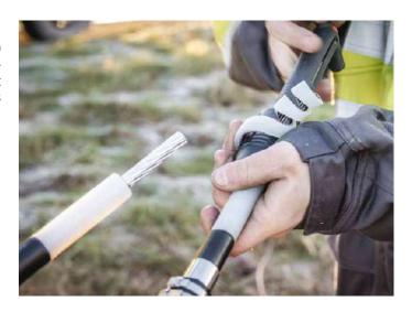
Ensto ST280 is designed to chamfer the primary insulation near the connector or lug in MV cables. This provides a smooth transition from insulation to connector or lug for the accessories installed. The application range ø is 15-60 mm and the chamfer is 45°.
