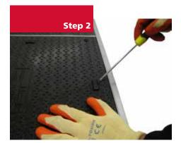
Remove the grommet on the closest side to where the operative is to remove the cover (Where the cover will be lifted to). Use a flat headed screwdriver to push under the head of the grommet until it wedges up.
