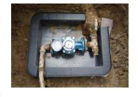
Sections can be cut on site to allow pipes to run through the chamber.
