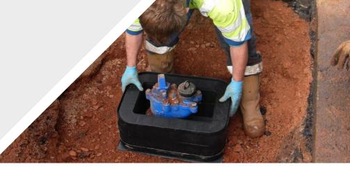
Developed specifically for use by water companies throughout the UK and Ireland, the STAKKAbox™ Water Chamber System offers an effective replacement to concrete sectional chambers.
