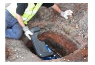
The chamber can be easily installed over existing valves using the split base.
