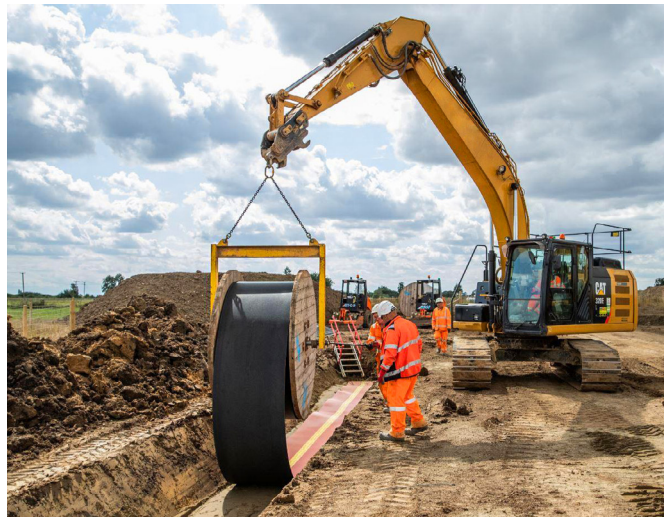
Installation of Stokbord® Drum at Triton Knoll Wind Farm
