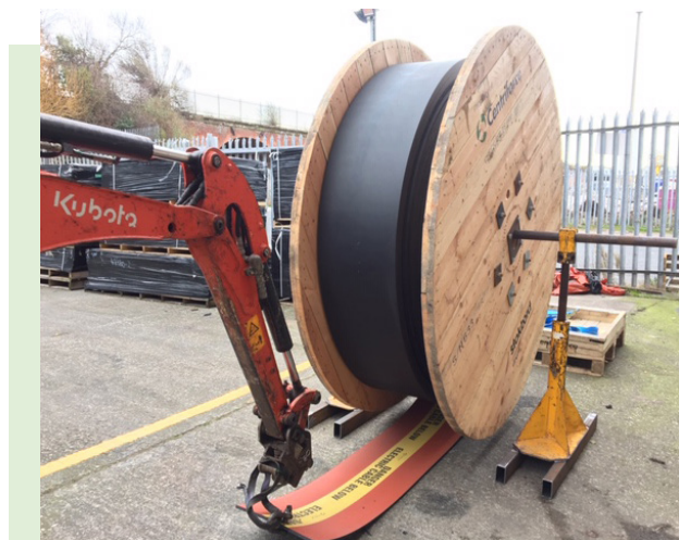
Stokbord® Drum mounted on screw jacks
