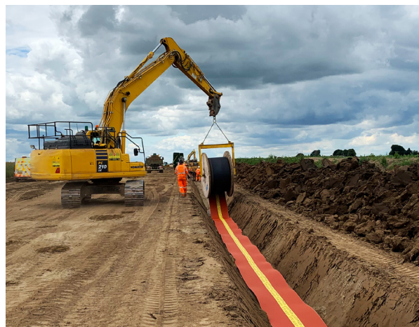
Excavator driving Stokbord® Drum into place
