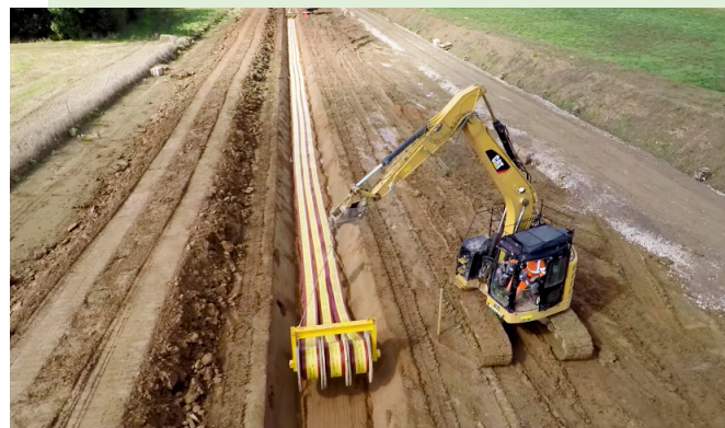
Laying Stokbord® Drum at Hornsea
