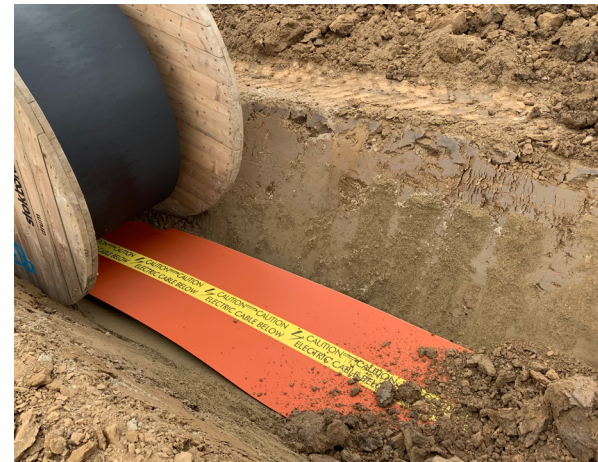
Stokbord® Drum held in place with backfill
