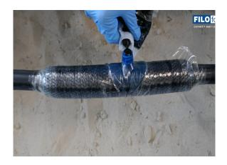
The FILOSLIM Cable Sheath Repair Kit utilizes a totally enclosed mix-and-pour polyurethane resin technology, designed for use as a permanent repair of damaged cable sheaths.
