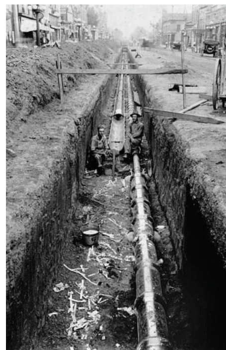
Figure 5 – Pipe laying in 1880, unencumbered by a proliferation of other buried utility services, and health and safety legislation
