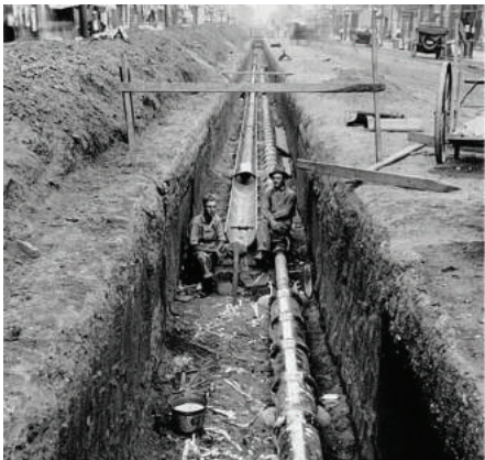
Figure 1 - An Old Problem, Still in Place: Open-Cut Trenching – Left: Laying of Sewer Pipe, Early 1900s (Courtesy of www.sewerhistory.org ) - Right: Utility Streetworks using Conventional Trenching, 2016
