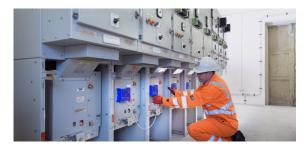
The **Astute® HV Monitor** is part of the award-winning **UltraTEV®** range. It is an advanced asset monitoring system for 24/7 monitoring of PD activity in all substation electrical assets. The **Astute® HV Monitor** is a modular system with up to 300 sensors that can be located across a switchboard to offer optimised coverage – typically without an outage being required.
