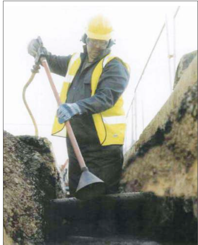
Figure 7 Using an air digging tool
