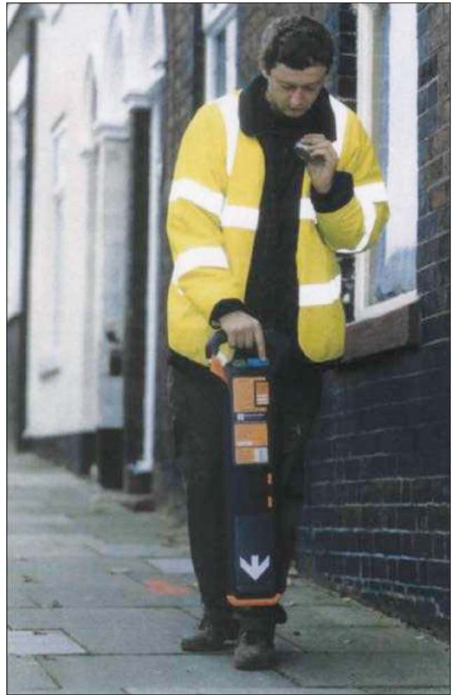
Figure 5 Using a cable locator
