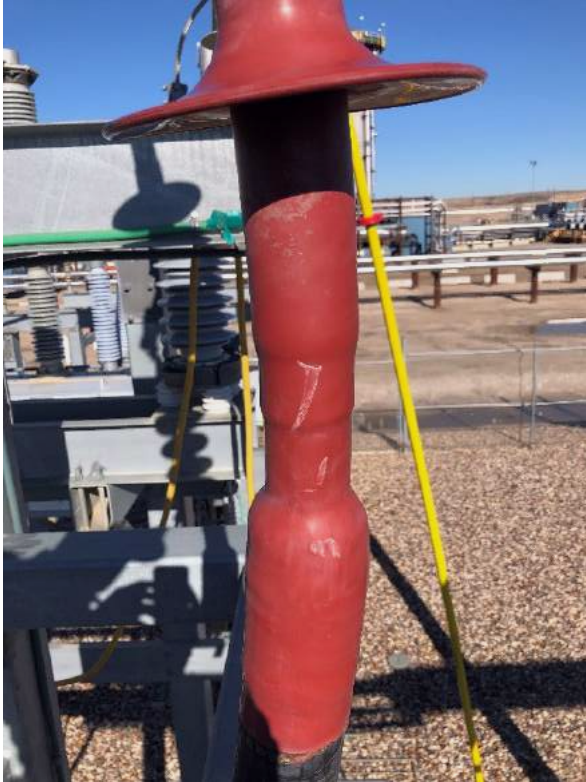
Cable termination H3 after cleaning
