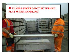
9. Products should be placed on a pallet in the same way they were delivered. With panels on their edge not flat on the pallet. All products are to be placed on the pallet and not dropped.
