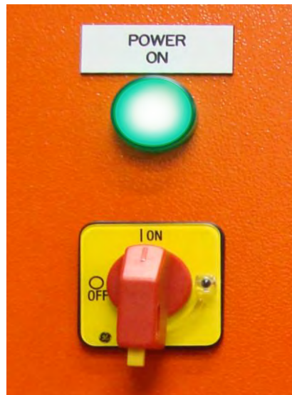
Figure 1-13: Main Power Disconnect
