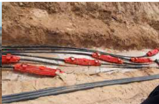
Straight through joints high water table
