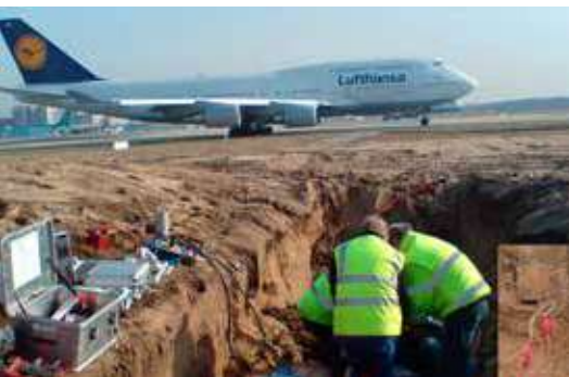
Transition joints Airport
